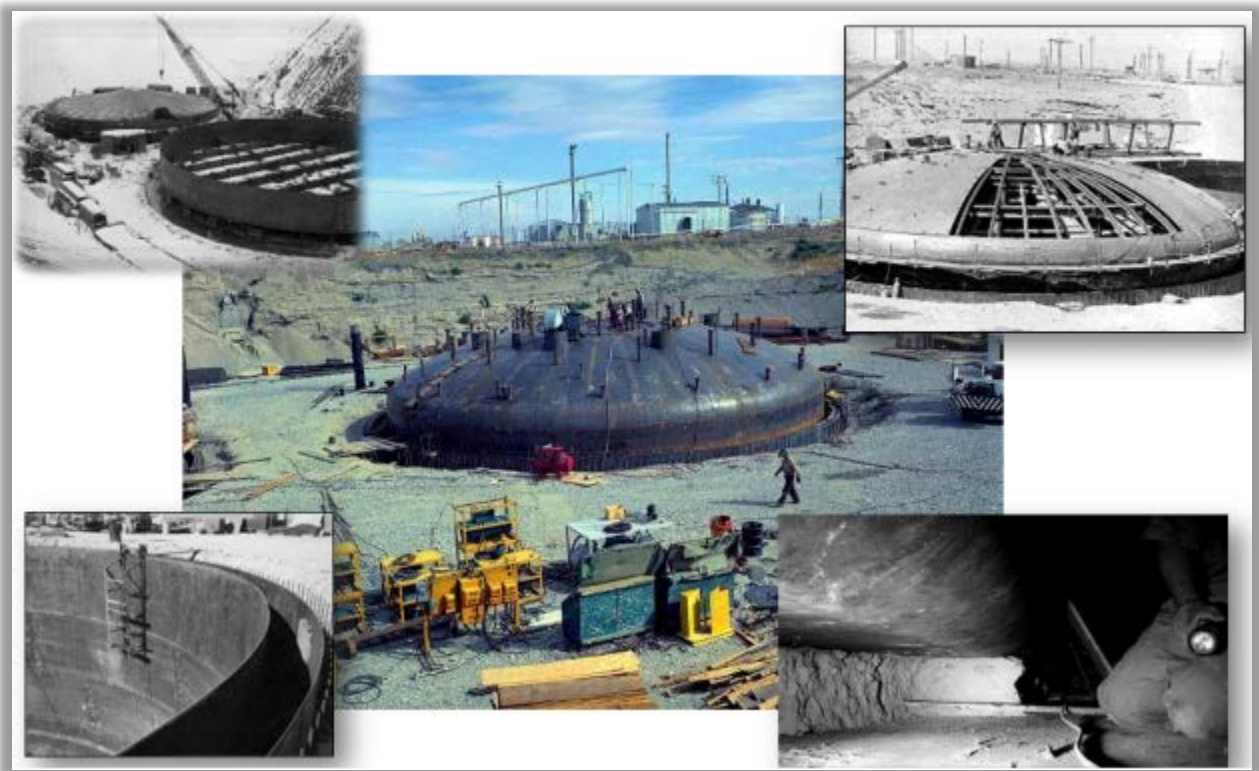
Figure 1. AY-102 Tank Construction
