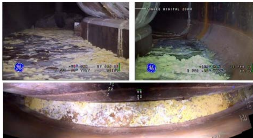
Figure 4. AY-102 Annulus Waste Accumulation 1
