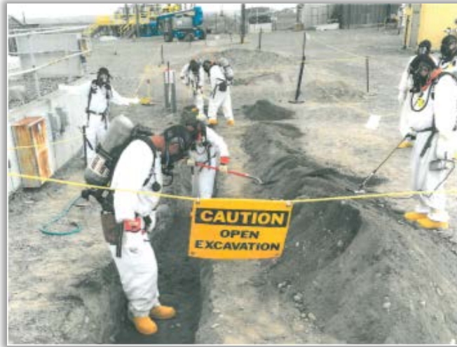
Figure 6. Trench Digging through 241-AX Tank Farm
