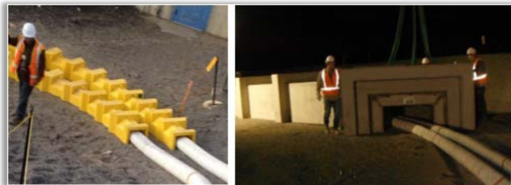
Figure 9. Lead-Antimony (left) and Concrete (right) Transfer Line Shielding Installation
