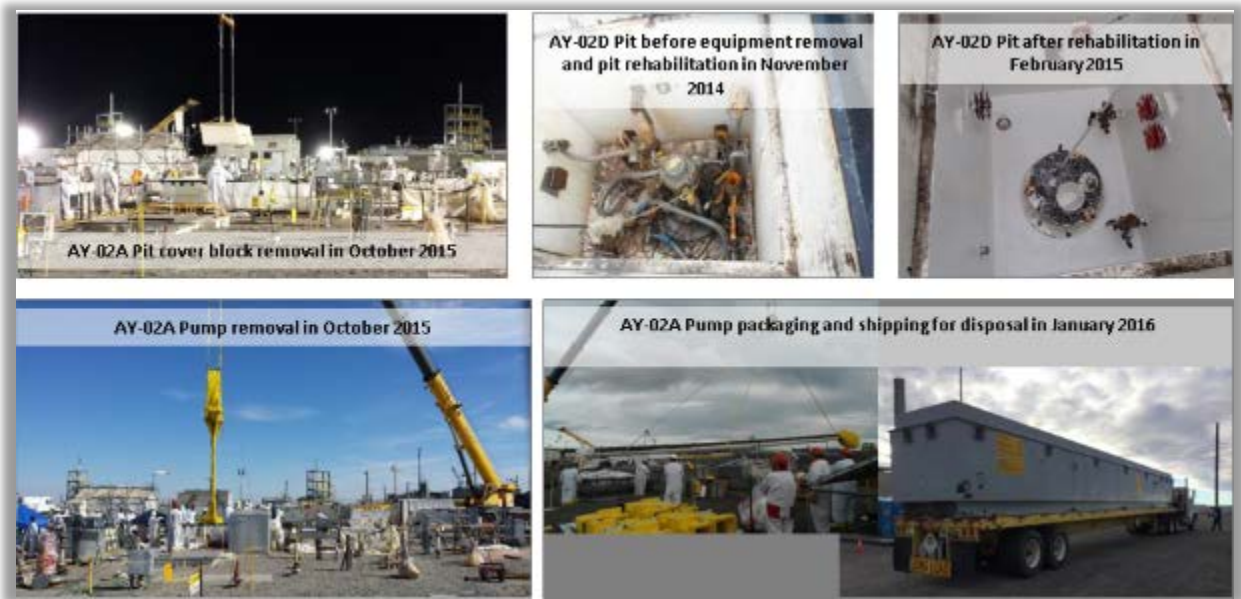
Figure 10. Tanks AY-102 and AP-102 Equipment Removal and Pit Refurbishment
